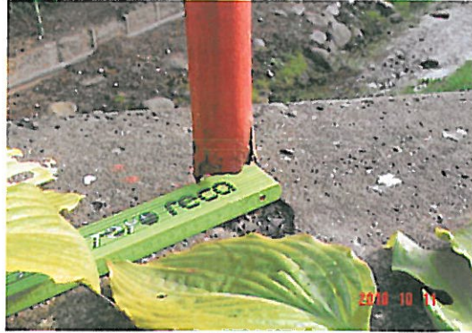
FUSS DES PFOSTENS DEFECT
